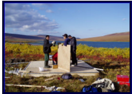
The floor of the tent frame is nearly completed.
