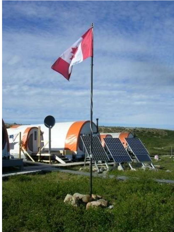
Photo 3: Weatherhaven buildings and solar panels at Daring Lake.
